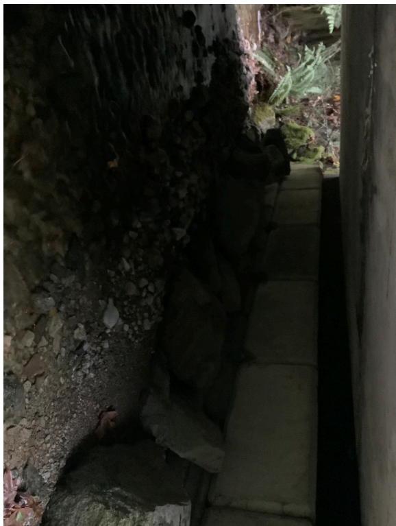
Right Bank Abutment when facing downstream
